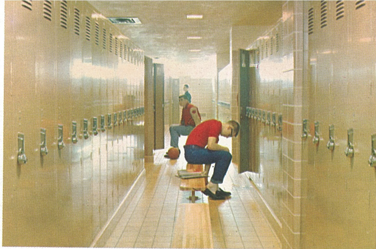
Locker room with 480 full-length steel lockers, each of which is continuously ventilated by an exhaust fan system in the floor. (A)
